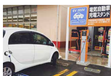
Began installing electrical vehicle charging stations
